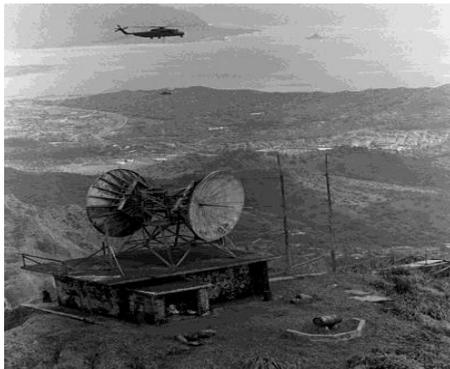
Fig.3. OMEGA Transmitter
